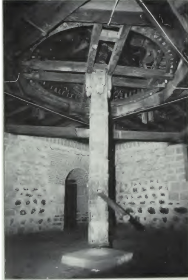
A. The mills were driven by mules that ploded around a capstan on the ground floor.
